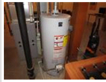
The average life expectancy for the hot water heater is 10-15 years, this unit is 8 year(s) old.
